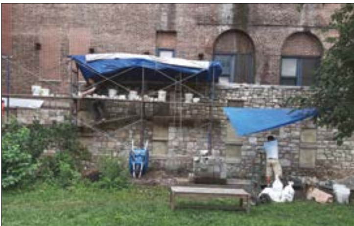
Stonemasons rebuilding north wall
