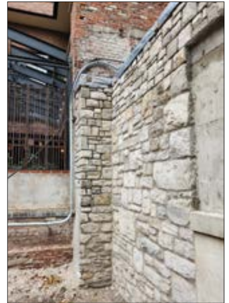
Finished corner October 2022
